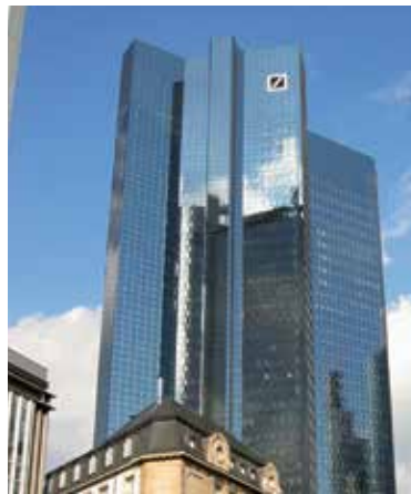
Location: Frankfurt, Germany Project: Deutsche Bank Application: AB-QM for Heating and Cooling
